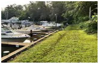
**Paths and Walkways.** The Deep Creek pier area also has a pier section between bulkhead sections with armor stone revetment that was recently replaced and appears in good condition. Along the bulkhead are wood walkways and a section of gravel path. The wood walkway appears in fair to marginal condition, and the gravel path appears in good condition and does not extend the whole way along the bulkhead from the Deep Creek pier access road.
