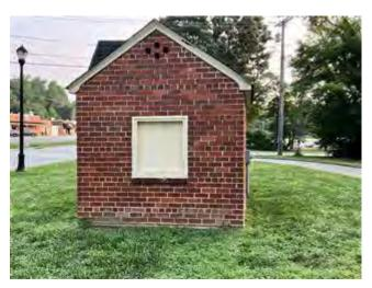
In general, masonry is considered a long-life item and is therefore excluded from reserve funding. However, because weather and other conditions result in the slow deterioration of the mortar in masonry joints, we have included funding in this study for repointing. Repointing is the process of raking and cutting out damaged sections of mortar and replacing them with new mortar.
