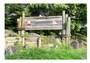
We recommend repointing and replacement of defective areas of the masonry as needed. The Association may consider applying a coating of Siloxane or other appropriate breathable sealants to mitigate water penetration and further degradation of the masonry work. The Association may consider applying a sealer to the carved wood sign to mitigate water penetration and further degradation of the wood.
