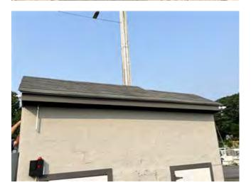
Asphalt shingle roofs can have a useful life of 20 to 50 years, depending on the weight and quality of the shingle. Weathered, curled, and missing shingles indicate they may be nearing the end of their useful life.
