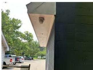
The Association maintains the exterior wood trim incorporated into the garage, gatehouse, and pumphouses. The Association may consider replacing failed trim sections with composite or capped PVC materials.
