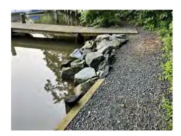
Stone revetments require a level of engineering design and permitting. Armor and Riprap stone revetments are designed to be durable and long-lasting. Permeable stone revetments, if properly maintained, can have a useful life of 30-50 years; however, proper upkeep of a stone revetment's annual maintenance will help it last decades and possibly a lifetime. The primary cause of shoreline revetment failure is hurricane storm surge, which can undermine the revetment.
