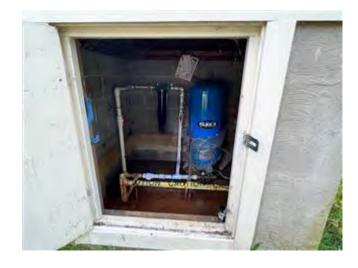
**Compressor Building.** The Association maintains a utility building at Deep Creek that houses an air compressor, electrical service, panels, security cameras, and a recorder. The building is constructed of cement block with an asphalt shingle roof and wood siding, trim, and doors that appear to be in fair condition.
