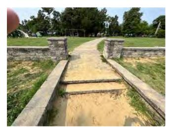
Segmental block retaining walls can have an extended useful life and, if stable, are likely to only require localized resetting of displaced blocks, typically near the top of the wall. This study assumes that resetting will be performed incrementally as needed. Segmental block retaining walls can have a service life of 80 years or more.
