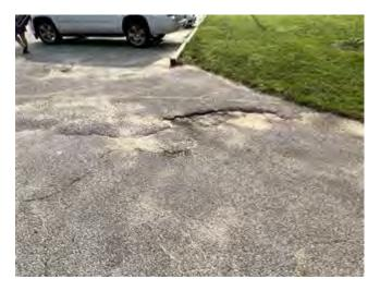
As a rule of thumb, asphalt should be overlaid when approximately 5% of the surface area is cracked or otherwise deteriorated. The normal service life of asphalt pavement is typically 18 to 20 years. Research has shown if installed correctly and with proper maintenance and seal coating the first year and every five years thereafter, asphalt pavement can have a service life of up to 40 years or more.
